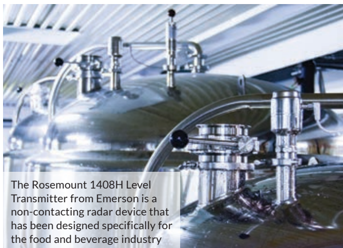
The Rosemount 1408H Level Transmitter from Emerson is a non-contacting radar device that has been designed specifically to provide highly accurate continuous level measurement in food and beverage applications
